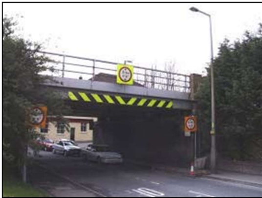
Photo: Typical layout of regulatory signs at a low bridge
