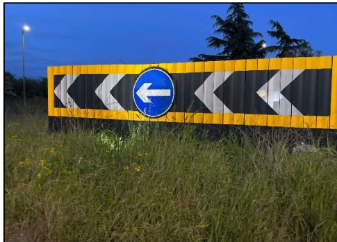
Photo: Prefabricated plastic chevron signs used on a roundabout
