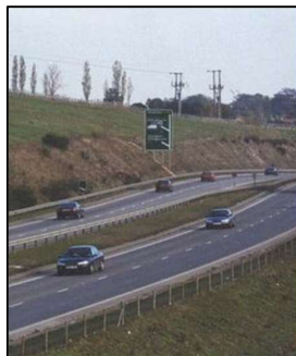
Photo: A sign mounted in a cutting or dip will reduce visual intrusion from the surroundings
