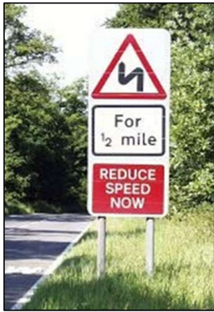
Photo: Appropriate use of grey backing board
