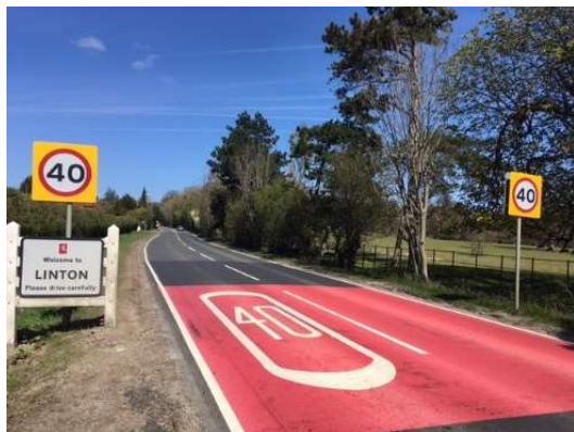
Photo: Red MMA surfacing used at a speed limit gateway
