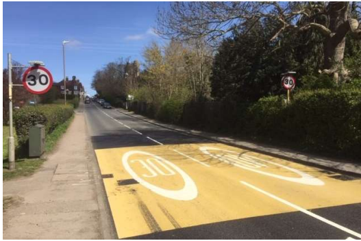
Photo: Buff MMA surfacing used inappropriately outside of a conservation area
