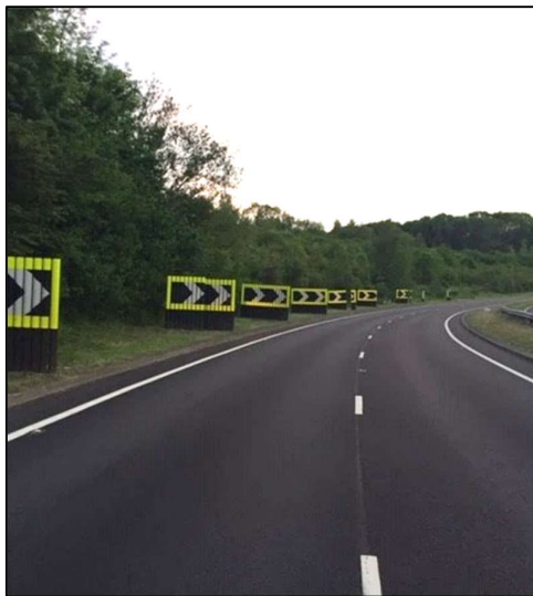
Photo: Prefabricated plastic chevron signs used to highlight a severe bend
